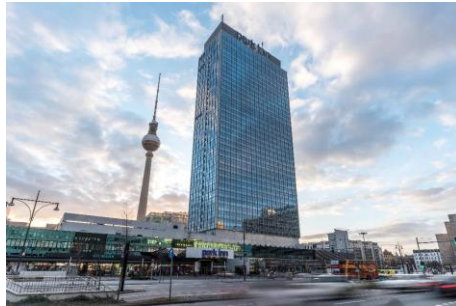
Park Inn Alexanderplatz
